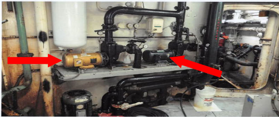
Figure 4.F. The above photo is of the two fixed bilge pumps located on the aft bulkhead of the lower engine room on the ALASKA JURIS. Date photo taken unknown.
